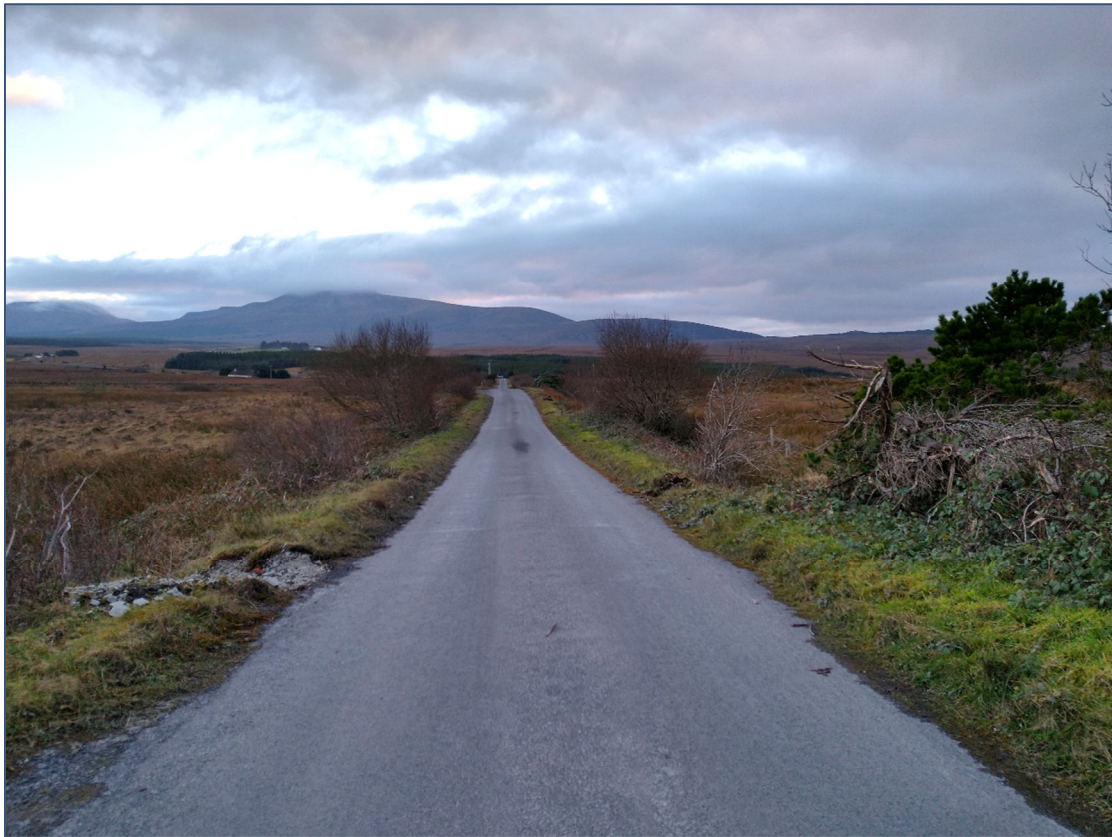
Plate 6-12: Existing road (BL3) into which the cable is going to be laid
