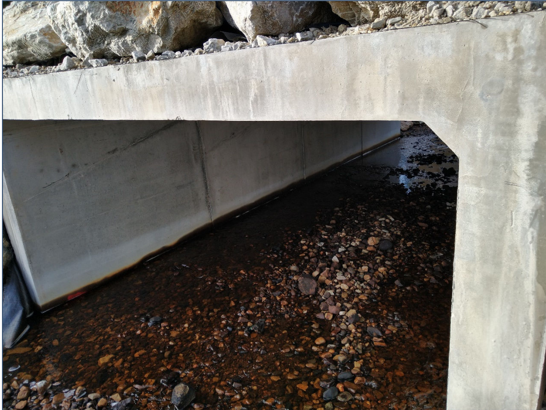
Plate 6-13 Example of an existing concrete box culvert crossing along the proposed access route
